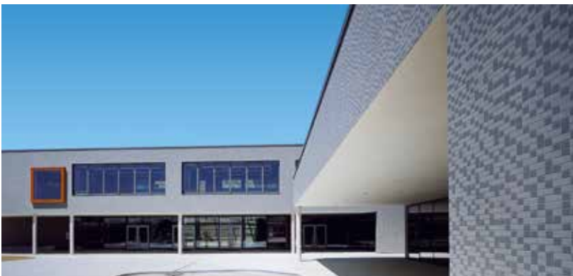
Elementary school, Erding/Germany Architectural firm: Dinkel, Persch/Stefan Dinkel, Munich/Germany StoVentec with ceramics
