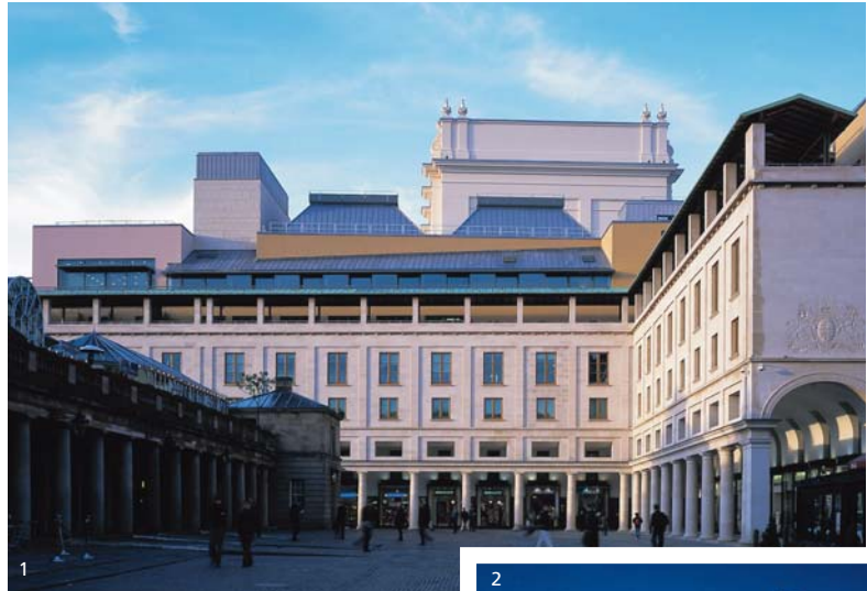
1: The Royal Opera House, London Architect: BDP Dixon Jones
