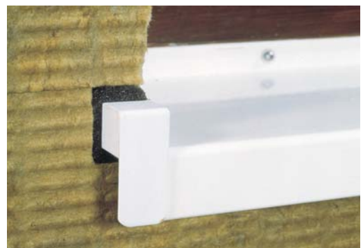
Special detailing around openings provides reliable weather-proofing.
